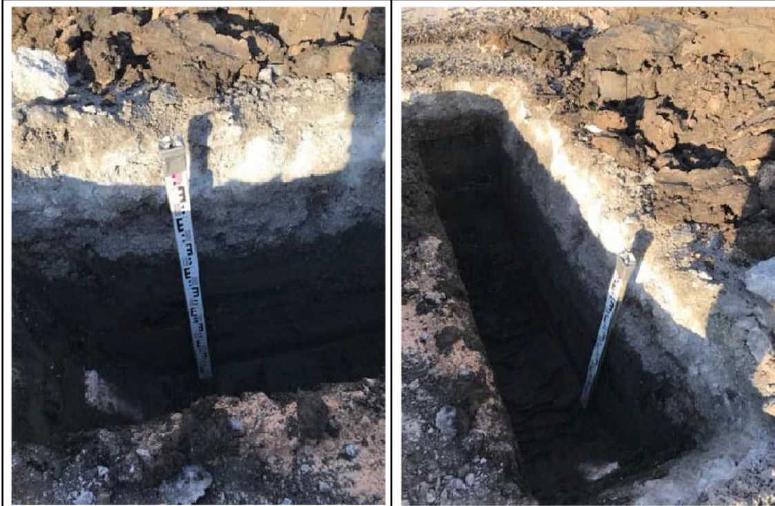
TP20 (Lean mix surfacing, subbase, landfill, alluvial Clay)
