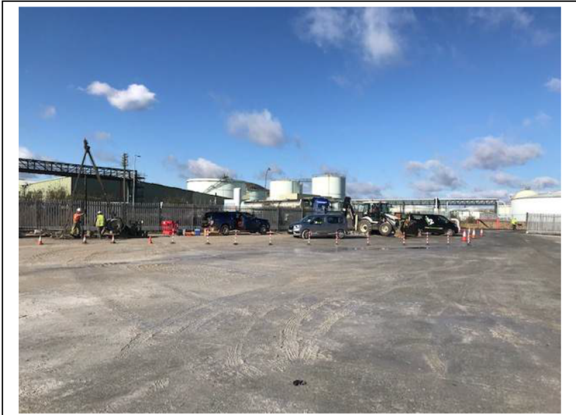
YARD 6, TP24 and BH05 with CBR testing underway
