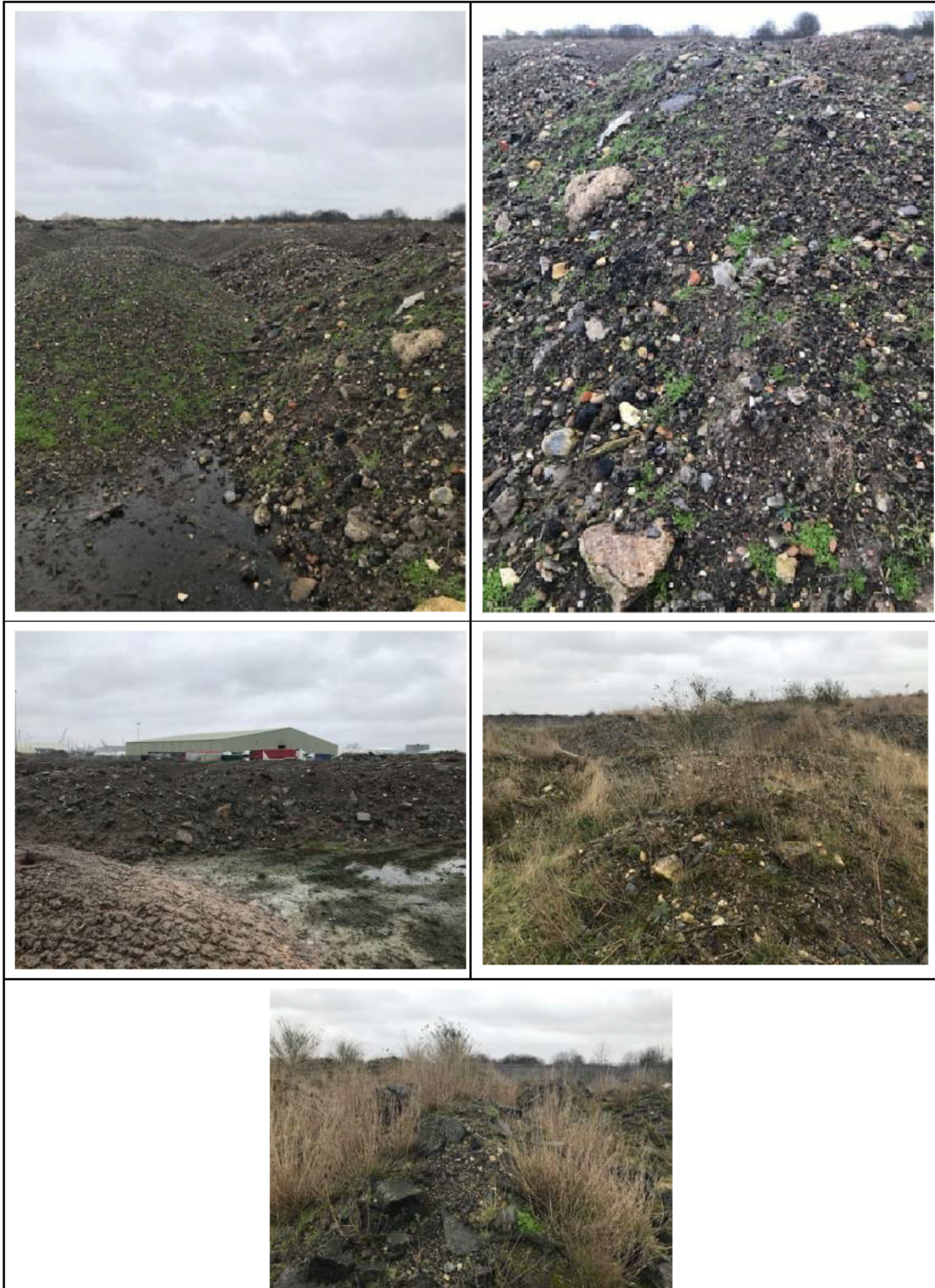
Area between TP08 and railway. Recent construction/excavation waste stockpiling. Large quantities of asphalt, kerbstones etc. Matrix is mixture of sands and clays, appears to be graded and possible crusher waste. Some very wet slurry tipping of unknown composition.
