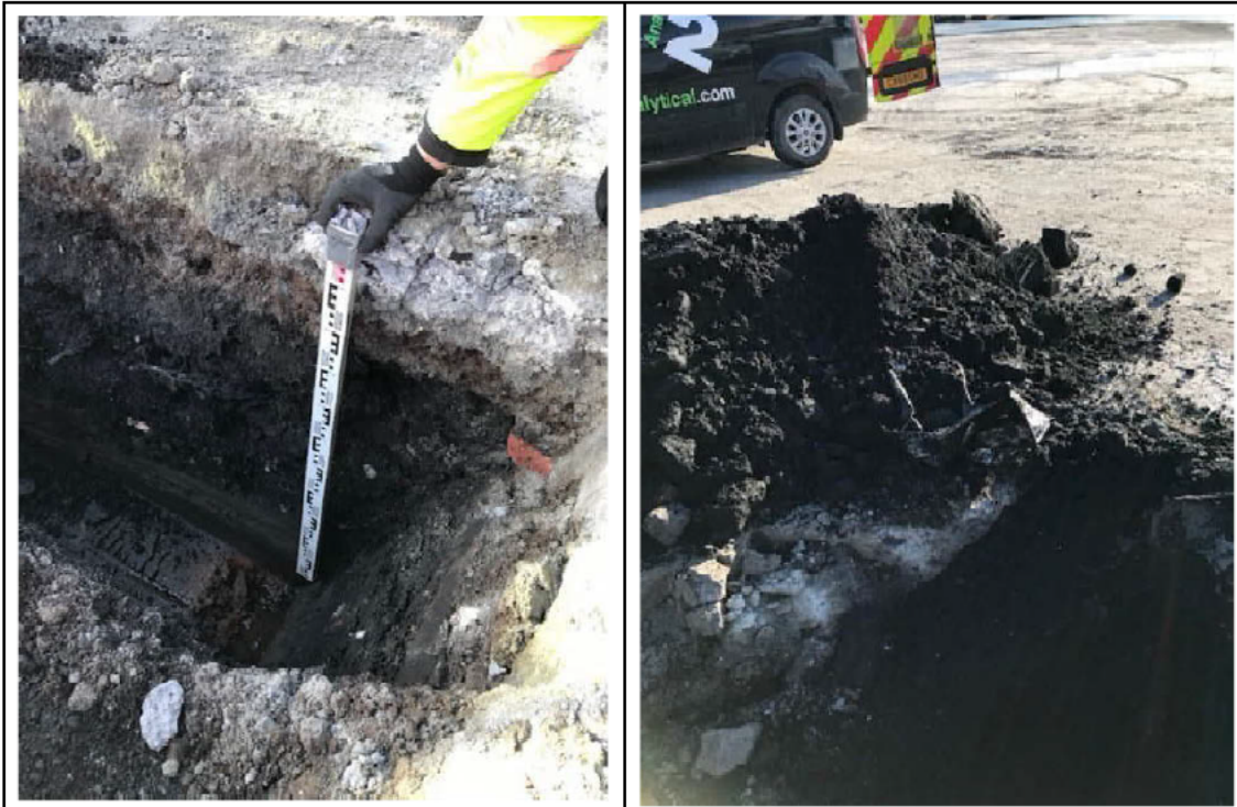
TP19 (Lean mix, subbase, landfill (including a sink, alluvial Clay)
