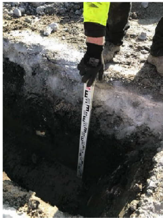
CBR at base of concrete/top of fill) 13%
