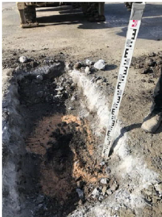
TP24 (Note: orange sand is from CBR test)
